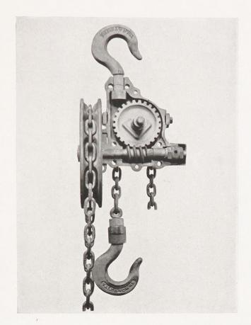
Half of housing removed to show bronze gear and steel worm-shaft
