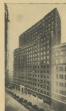
Bartholomew Bldg. New York City, N. Y. Archts.: Starratt & Van Vleck
