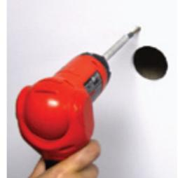
2 Drill holes into the drywall and insert the drywall mounts.
