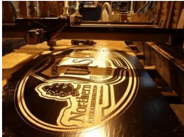
Pocketing of area between border and design in progress.
