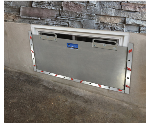
#5128MA mounted to a basement window.
