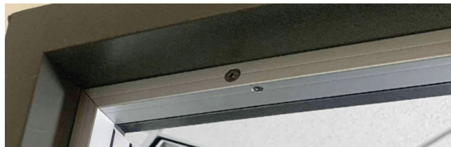
#5077CA Installed on head of frame.
