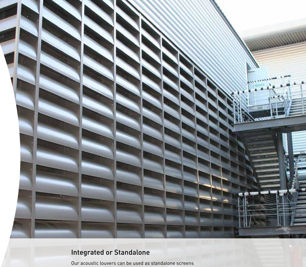
Our acoustic louvers can be used as standalone screens around mechanical plants, or be integrated into walls and building façades.
