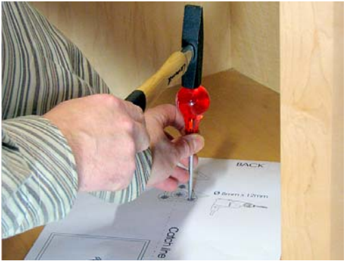
2. Mark the drilling holes
