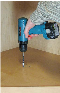
3. Drill at top and bottom (Ø 8 mm)
