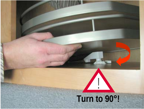
3. Putt the fitting in bottom bearing
