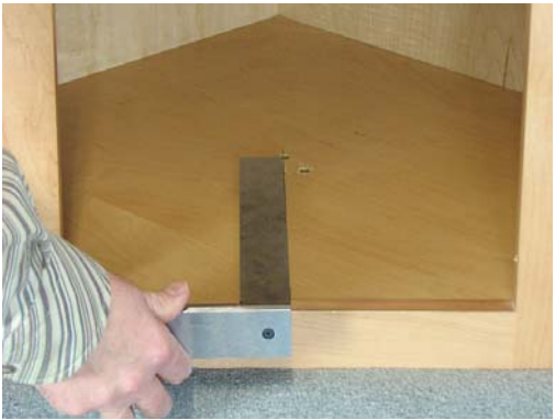
4. Makr the middle line at the bottom
