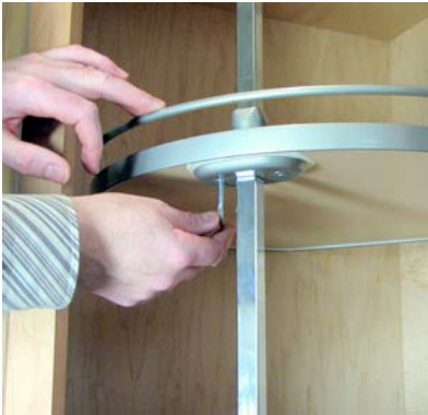
3. tight the upper shelf in the required height
