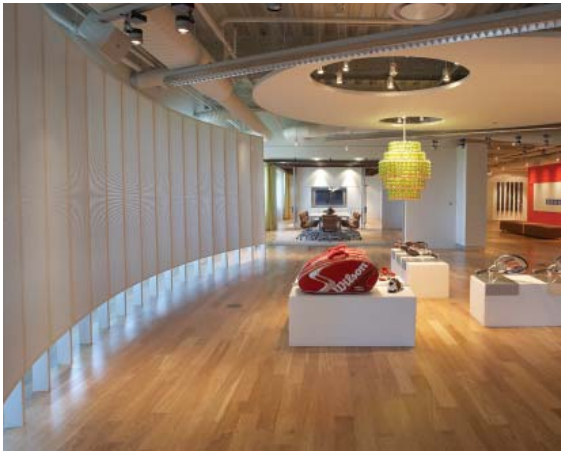
Fry Reglet Acoustical Wall Panels secured to aluminum posts are used as a projection screen at Wilson Sporting Goods Headquarters.
