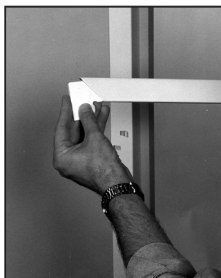
6 Slide corner backing angles into header casing.
