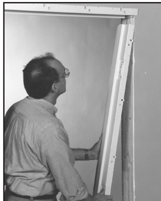
2 Set hinge jamb over wall section.
