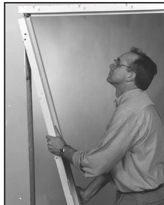
3 Set strike jamb over wall section.
