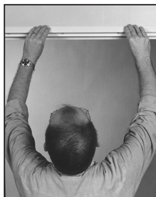
7 Snap on header casing.
