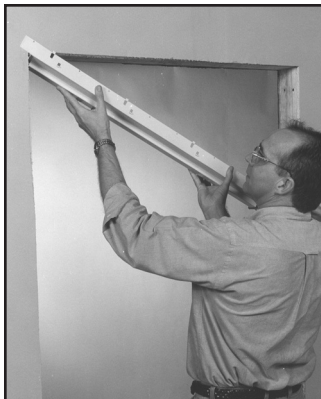
1 Set header over wall section.
