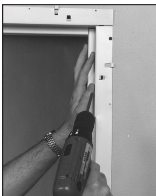
5 Apply fasteners starting at upper end of hinge jamb.
