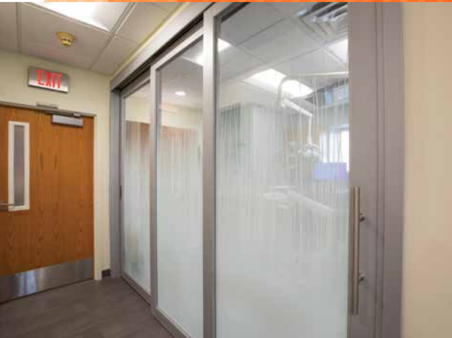
Sliding doors can create wide openings to better accommodate mobility-assistive devices.
