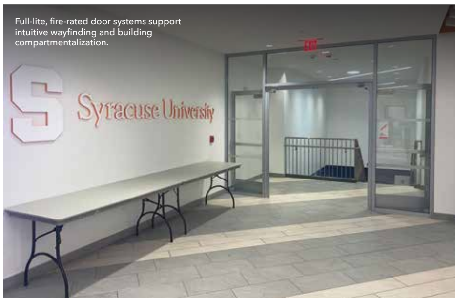
Fire-rated glazing meets code requirements without sacrificing design intent for a safe and welcoming built environment.
