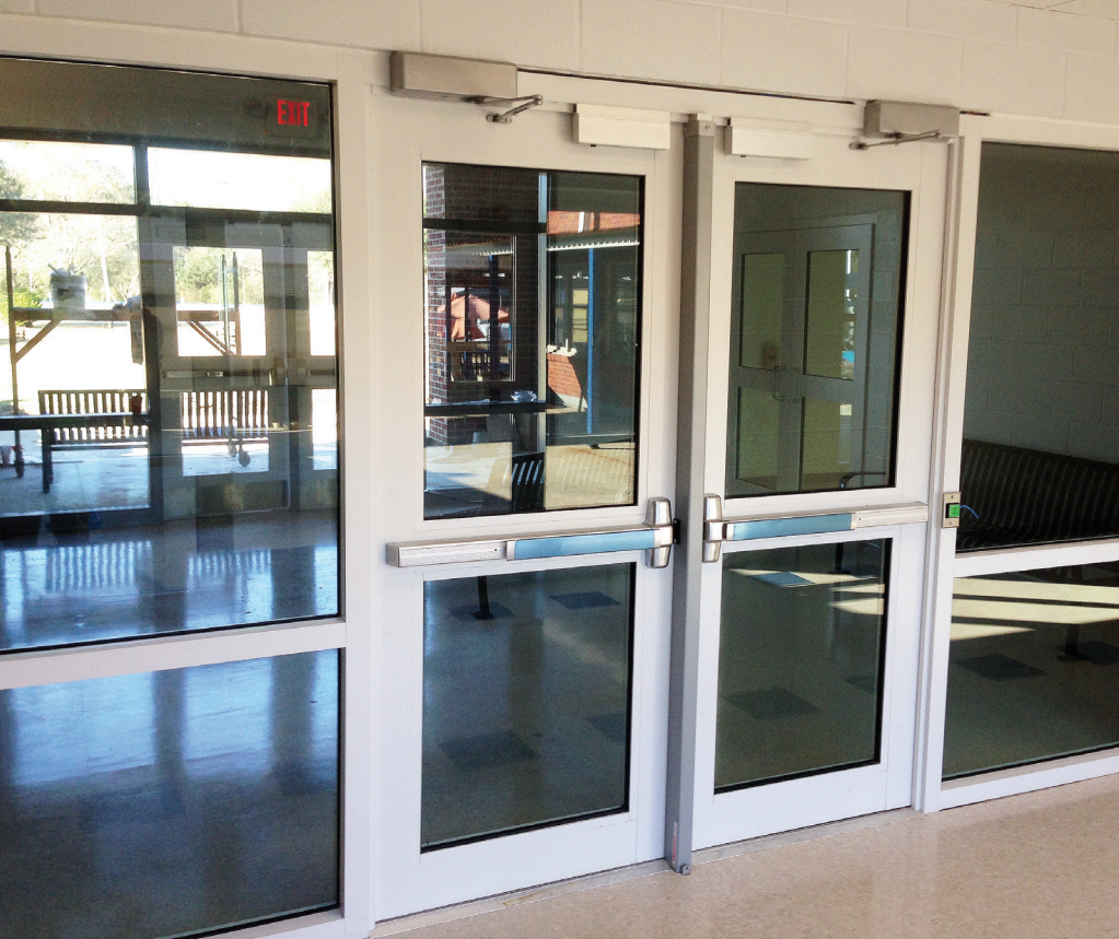
Aluminum doors with ballistic protection at Central Elementary School in Maryland.
