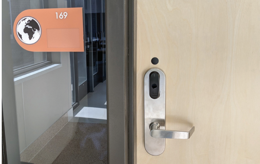
A wireless classroom lock is able to be locked down remotely.
