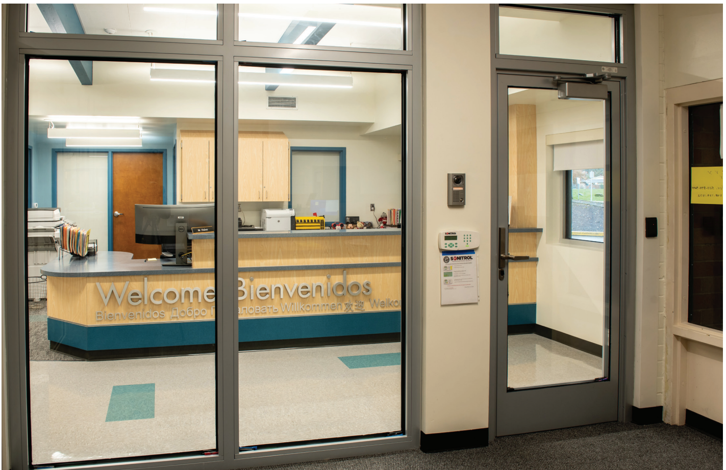
The fire and security solution at Candy Lane Elementary offers bullet-resistance rating and withstands forced-entry attacks.
