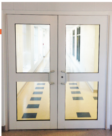
Aluminum doors with ballistic protection at Central Elementary School in Maryland.
