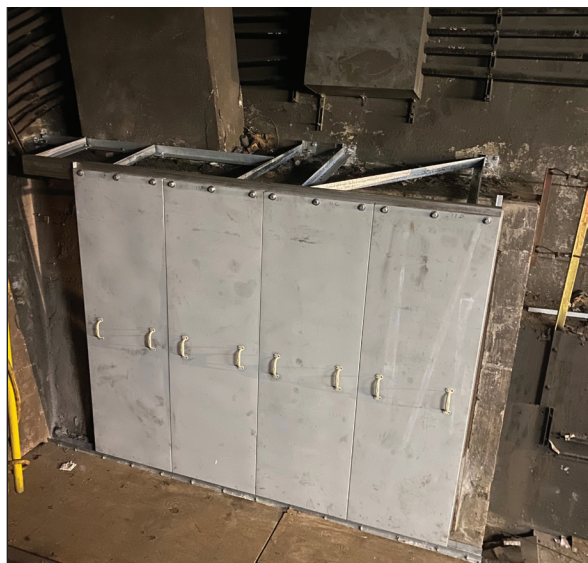
Access panel doors installed and awaiting final paint.
