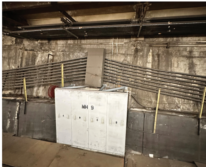
View of finished access panel doors installed in train tunnel.
