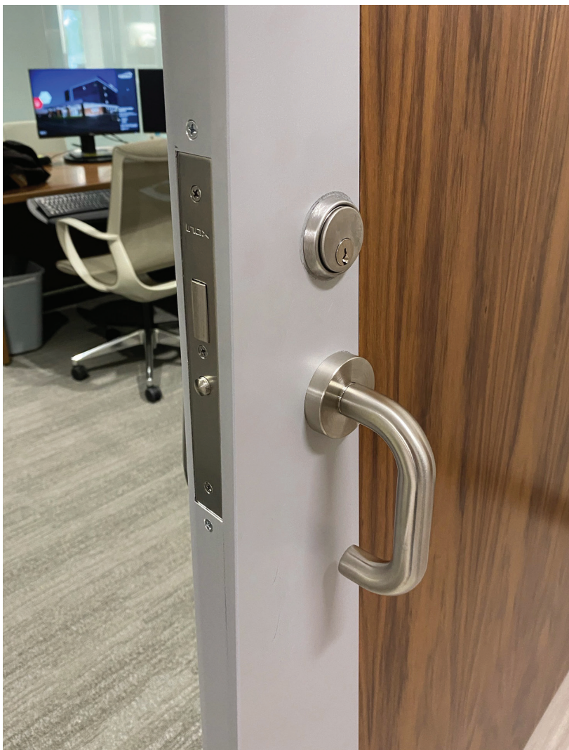
When the door is closed, the release button is activated, which triggers the deadbolt into the strike.
