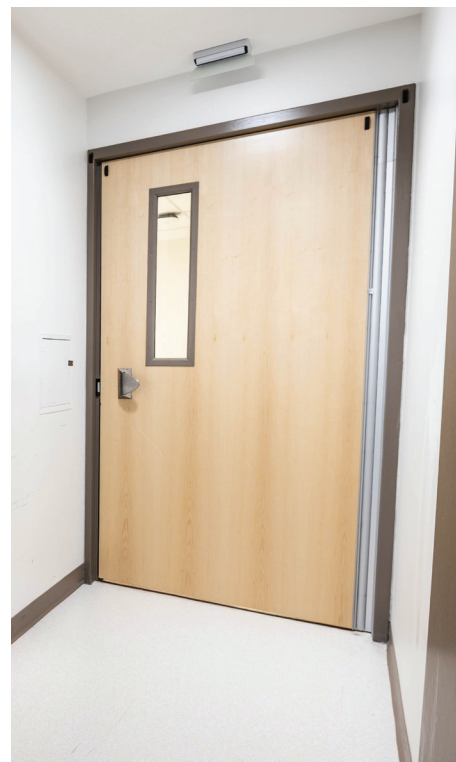
This door with double swing continuous hinges and emergency release stops eliminates the gap adjacent to the hinge, protecting patient privacy.
