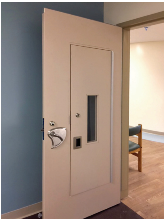
Behavioral health access doors give caretakers or authorized personnel quick access to a patient's room in case of an emergency.
