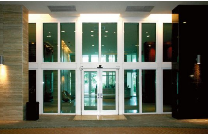
90-minute, temperature rise pair of doors with a clear anodized finish at Harvard Business School's Klarman Hall in Boston, Mass.
