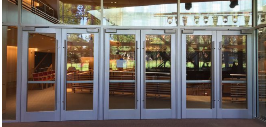
90-minute, temperature rise and hurricane rated pair of doors, Las Olas Beach Club, Ft. Lauderdale, Fla.
