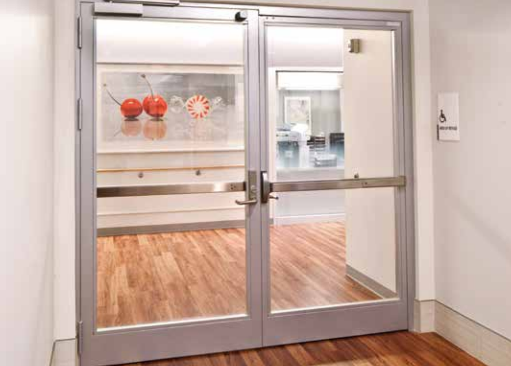
Steel doors and frames with glass ceramic, University Hospital, Seidman Cancer Center, Cleveland, Ohio
