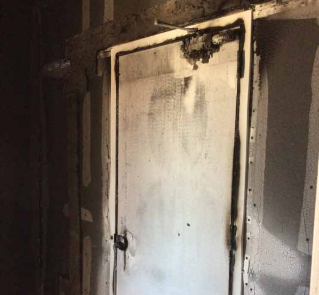
This door was burned from both sides hours apart and still stayed latched. What is normally a very heavy door turned into a what felt like a piece of balsa wood in weight.
