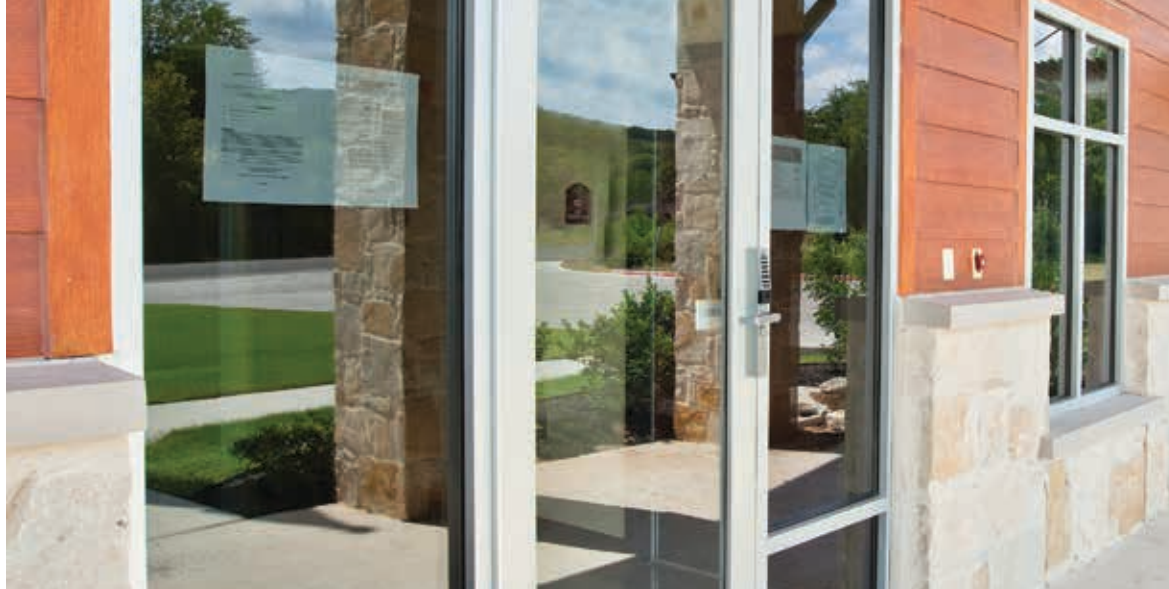
At a fire station in California, a push-button lock allows quick access to fire fighters who know the PIN, but guards the entrance when the station is unmanned.
