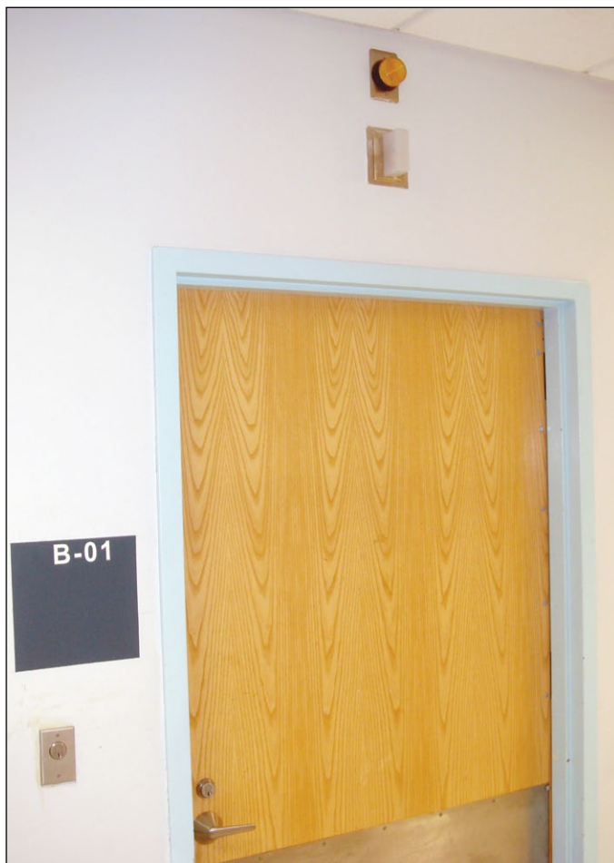
Exterior view, including lockset, key reset switch, and strobe for alarm (strobe is above nurse call light).
