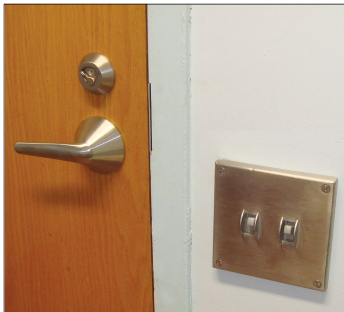
Privacy function lockset with ligature-resistant lever and turnpiece. Light switch with ligature-resistant elements is also shown.
