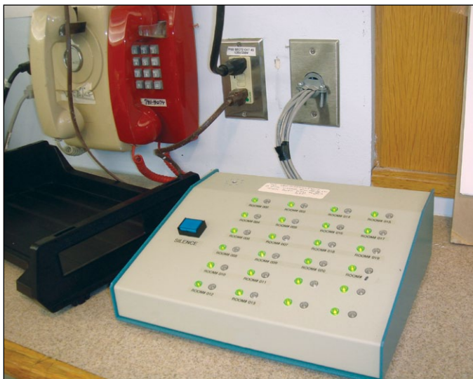
Nurse's station for door notification alarm with illuminated LEDs showing fully-monitored position of each activating bar. Individual red LED illuminates in emergency condition. Local momentary silence switch is on the left.
