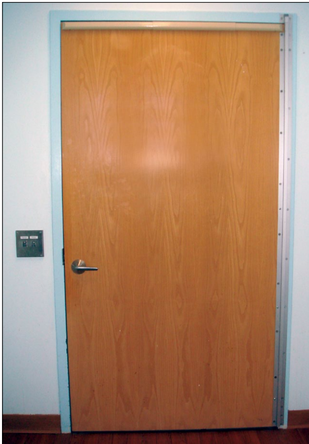
Interior view of a typical patient room door with ligature-resistant items, including lockset, hinge, light switch, and door notification alarm activating bar across the door
