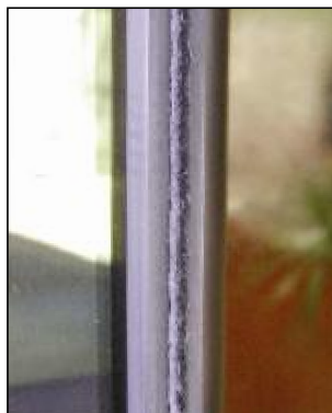
Press new pile into groove with screwdriver
