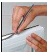
Remove old pile from frame
