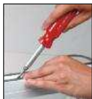
Press new pile into groove with screwdriver
