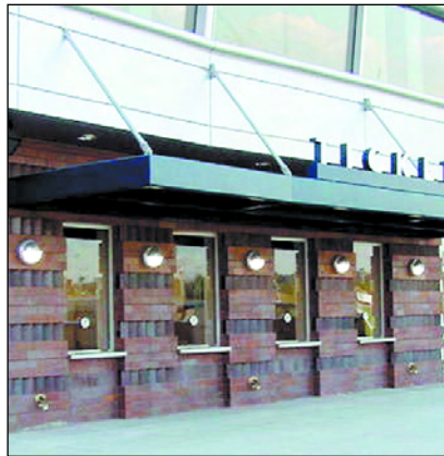
INVESCO Field, Denver, CO. Installation by A-1 Glass Inc.
