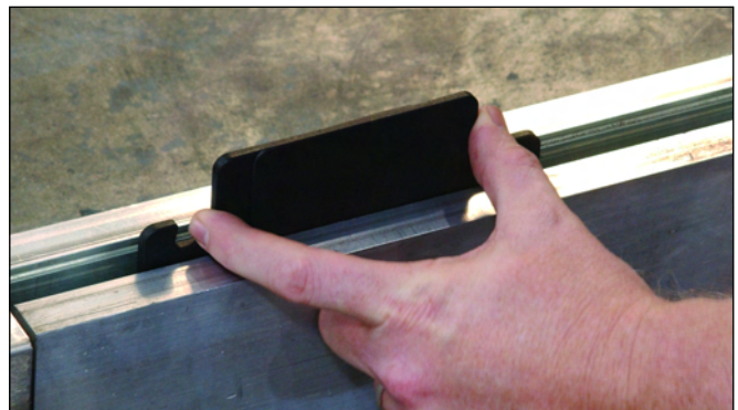
Install the TAPER-LOC™ Tapers Finger Tight into the Base Shoe
