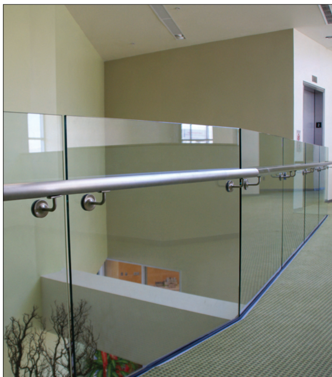
Glass Mount Brackets With Hand Rail Tubing
