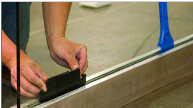
Install the TAPER-LOC™ Tapers Finger Tight into the Base Shoe
