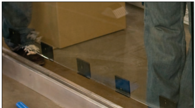
Installing the L-Pressure Block on the Bottom Edge of the Panel and Setting the Panel in the Base Shoe
