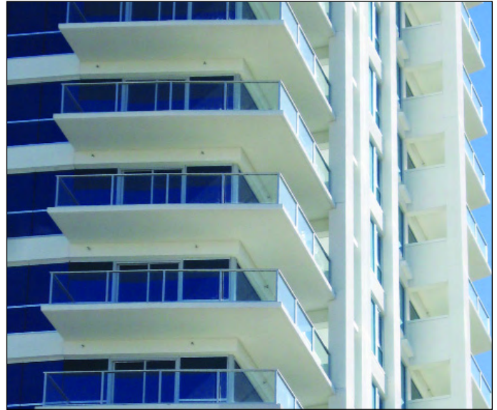
ARS 350 Series Aluminum Railing System With Glass Infill
