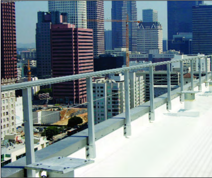
ARS 200 Series Aluminum Railing System With Cable Infill and Fascia Mounts
