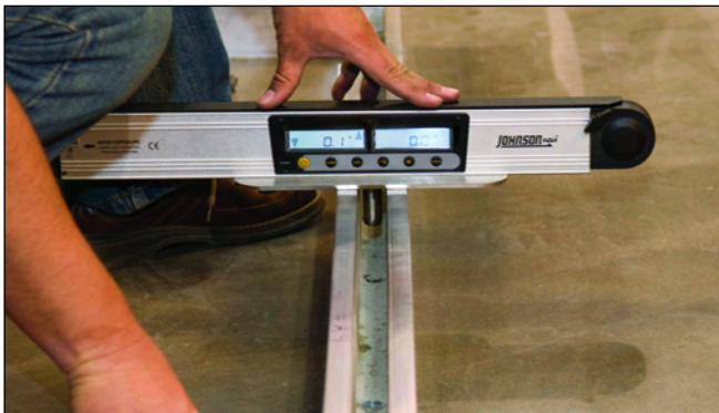
Leveling the Base Shoe Using Our PAL1K Plumb/Angle/Level Locator Kit
