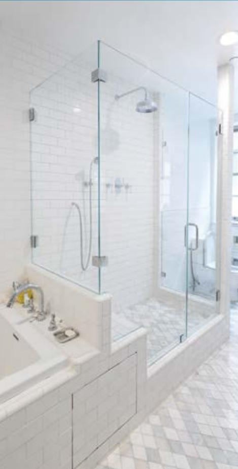
Many CRL Hinges utilize the same cut-out in the tempered glass. This is by CRL's design. It not only allows you to present options to your customers when choosing the particular model of hinge for the job, but also allows an opportunity to go back later and re-install a different hinge in the same cut-out, should a customer make décor changes. This page shows you the different hinge groupings which share the same glass cut-outs.
