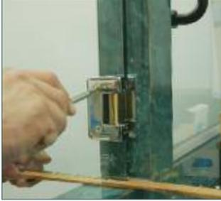
Loosen the cover plate and align the door.
