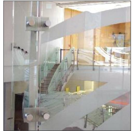
CRL's 1-1/2" (38.1 mm) Diameter Standoffs are perfect for attaching heavy glass, granite, and marble to the top of cabinetry. They are available in Brushed or Polished 316 Stainless in a range of standard lengths from 1/2" to 4" (12.7 to 101.6 mm).
