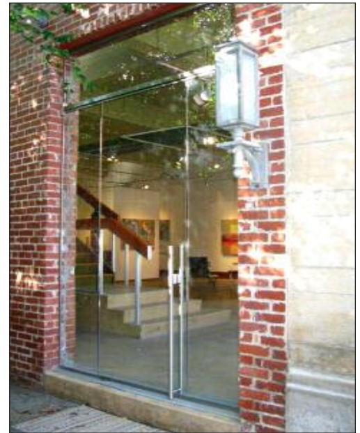
Mechanical Glazing Channel used on perimeter verticals and above transom.
