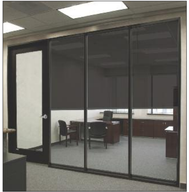
Offset Glazing Allows for Window Coverings
