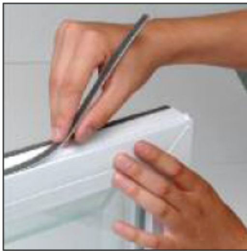
Remove old Pile from frame
