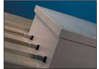
Curb Modification for Metal Buildings
