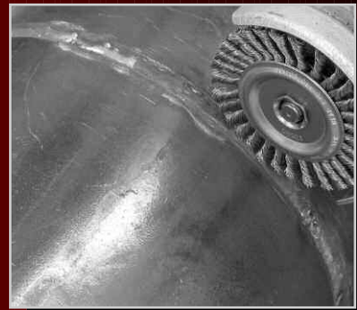
Weld cleaning with a stringer bead knot wheel. This brush offers a narrow face width and aggressive brushing action for fast, efficient use in weld cleaning such as the pipeline application pictured.
