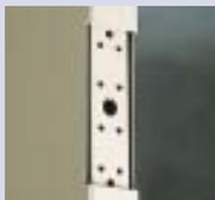
Standard Non-handed hinge preparation. (minimum 10 gauge). Prepare for standard and heavy weight 4.5" Hinges
