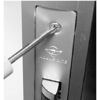
Fig. 5e: Install the latch face plate
