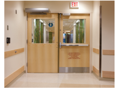
In the 2015 edition of the IBC, the activation time for delayed egress locks was changed from 1 second to 3 seconds, which is consistent with NFPA 101.
