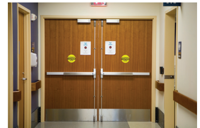
Controlled egress locks are allowed in some health care units, but staff must be prepared to facilitate egress if needed.
