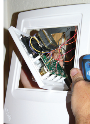
Figure 8 - Placing Room Station in
