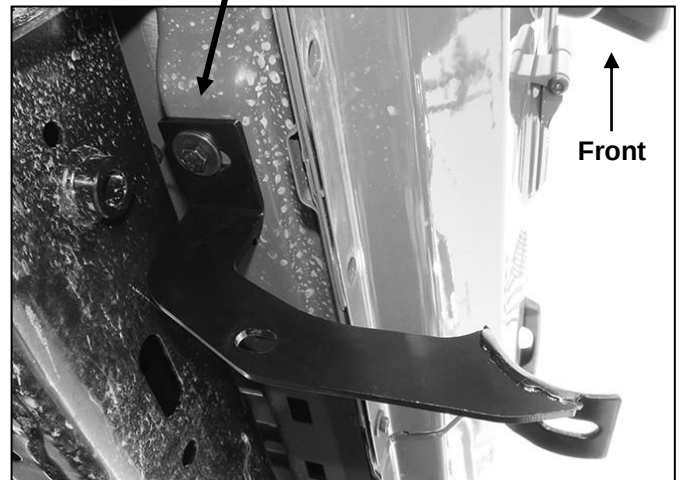
(Fig 4) Driver/left front Mounting Bracket installed
