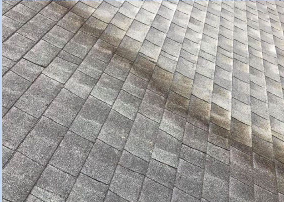
Asphalt shingle roof, before (bottom left), after (upper right)
