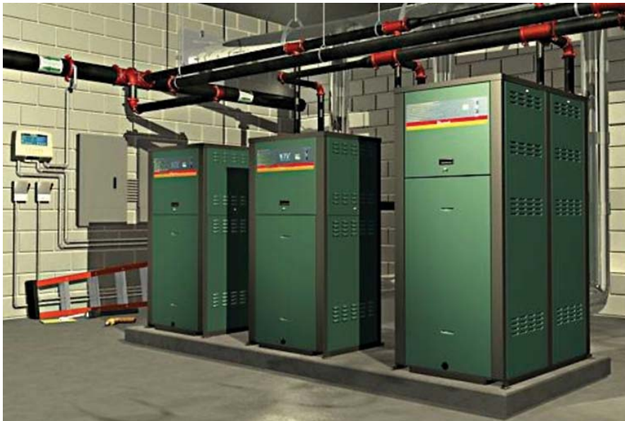
A hybrid variable-primary-flow system with wall-mounted sequencing controller plumbed for primary/secondary pumping using one condensing boiler and two non-condensing boilers.
