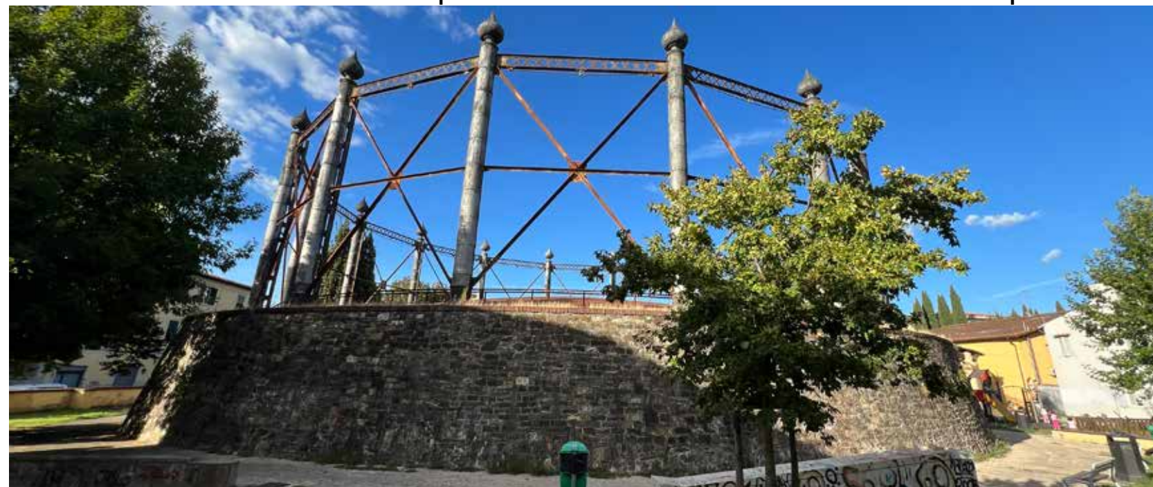
gasometer on site
