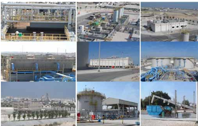
Bapco's Waste Water Treatment Plant
