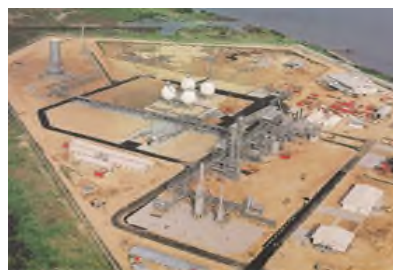
Photo by Chevron Onshore Escravos gas plant, helps to utilize Nigeria's gas potential and eliminate gas flaring.
