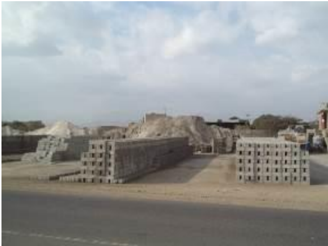
Plate 4.3: Cement Block Manufacturing Unit
