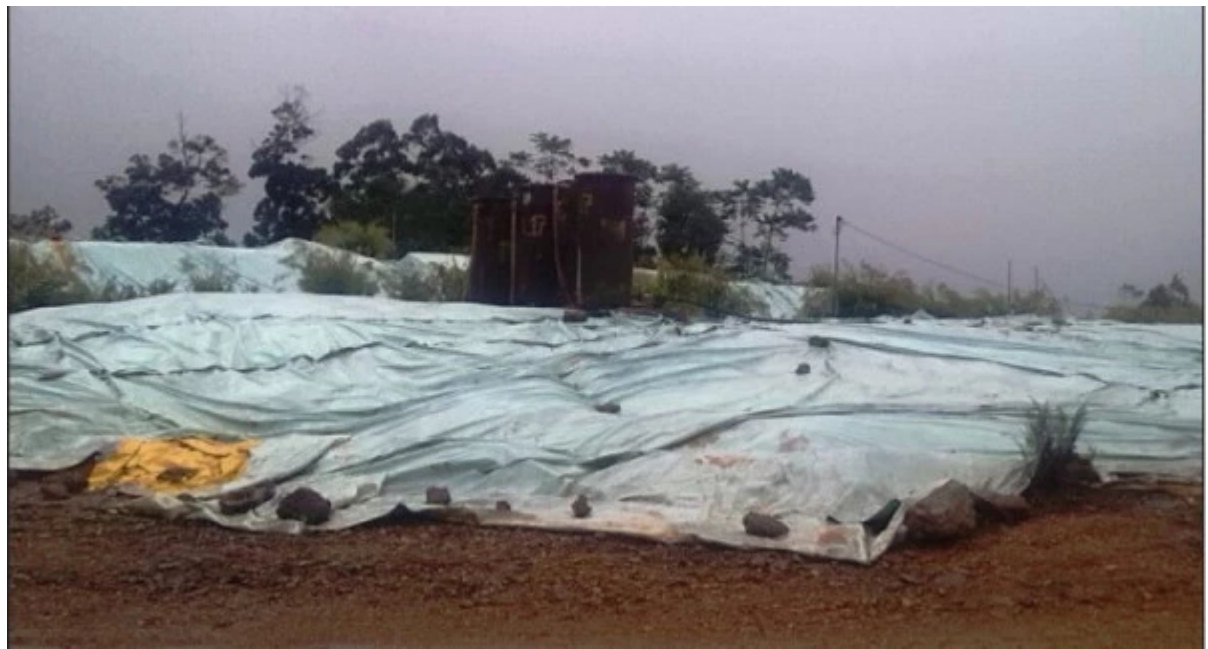
MRA allowed New Guinea Gold to abandon the Sinivit mine in 2014
