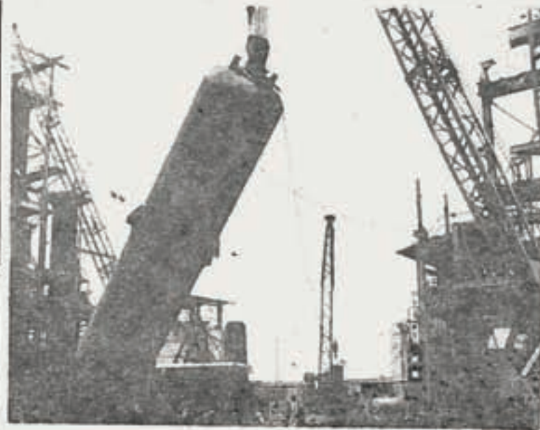
120 TONS OF STEEL COMES GENTLY TO EARTH as the B. J. Project team lower one of the disused coke chambers on the Thermal Crackers preparatory to moving it to the site of the new Platformer. There it will be used for hydrogen storage.
