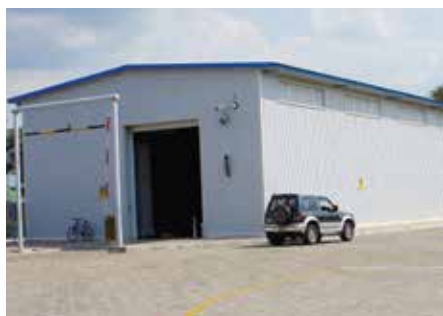
The Scanning Hall at Tlokweng Gate Border
