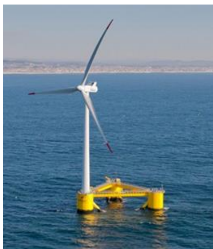
Full-scale prototype of WindFloat device.
