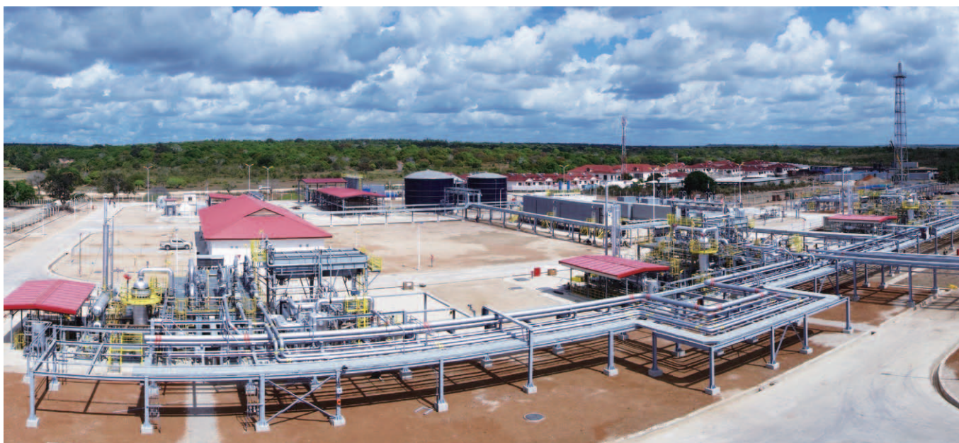
Gas processing plant in Tanzania
