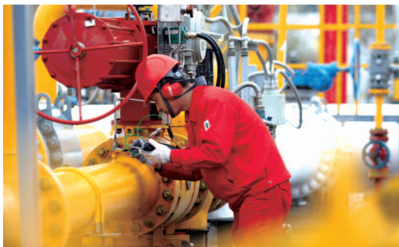
Routing inspection at gas station
