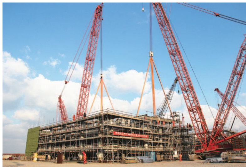
Construction of MWP4 engineering package of Yamal LNG project
