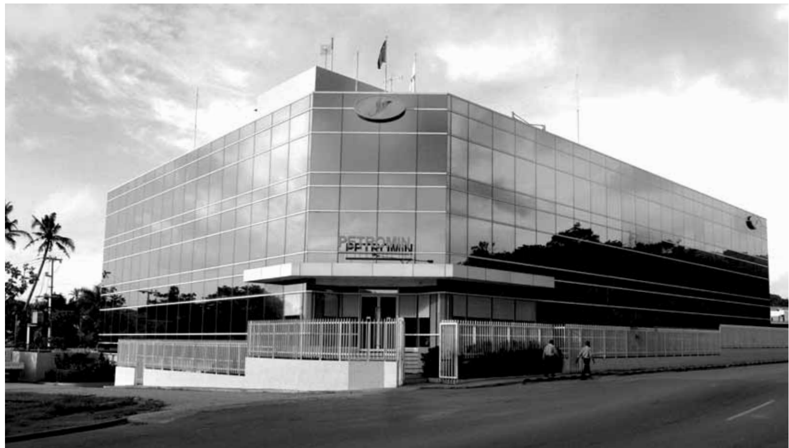
Petromin Haus located along the Sir Hubert Murray Highway
