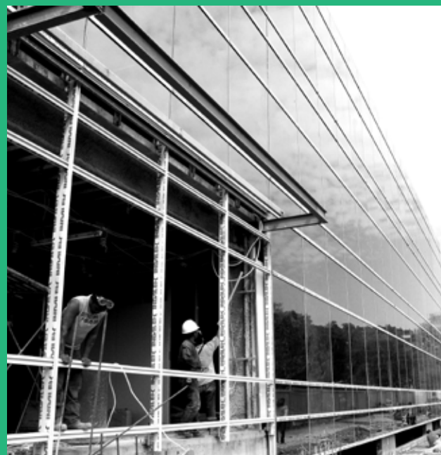
Construction of Petromin Haus
