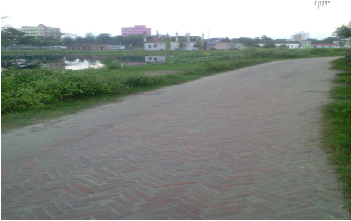
RCC Palisading work with earth filling beside Mizmizi TC road to Dhaka-Chittagong highway via main road.
