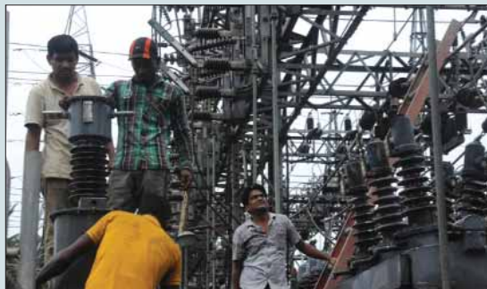
Technicians tried to repair at Katakhal grid sub-station people of Rajshahi region get electricity from this sub-station
