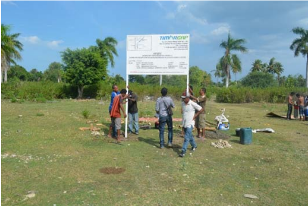
Site survey and placard installation for the fuel stations
