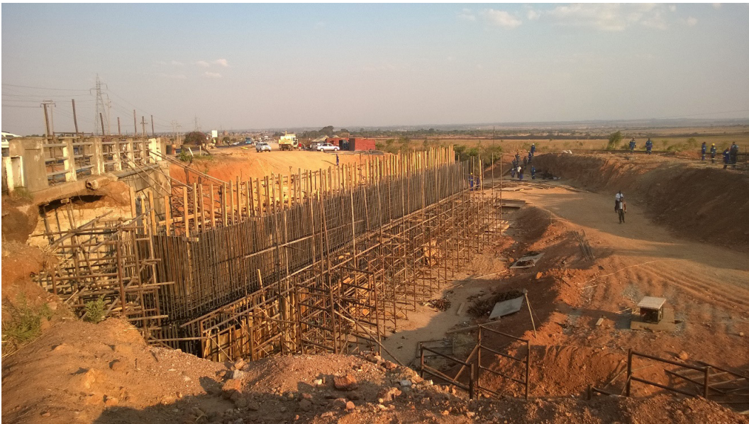
Mabvuku road over rail bridge
