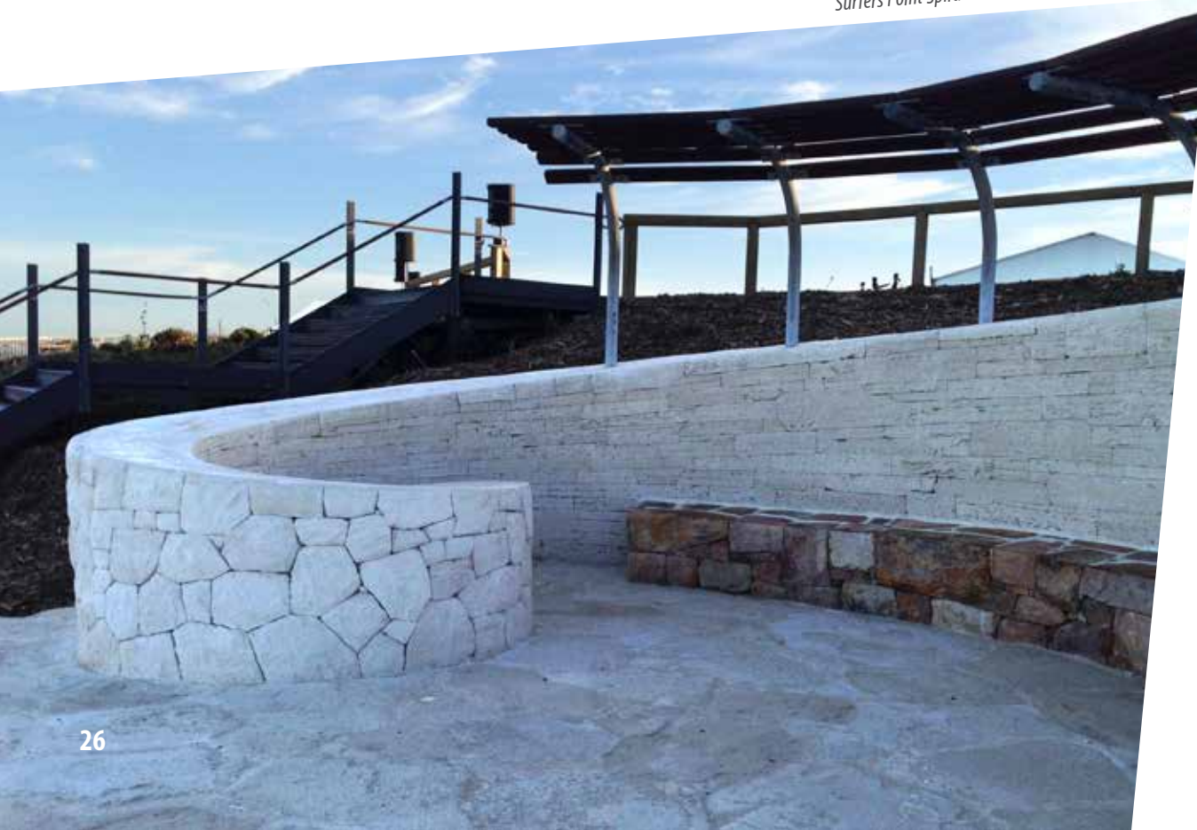
Surfers Point Spiral Shelter, Margaret River
