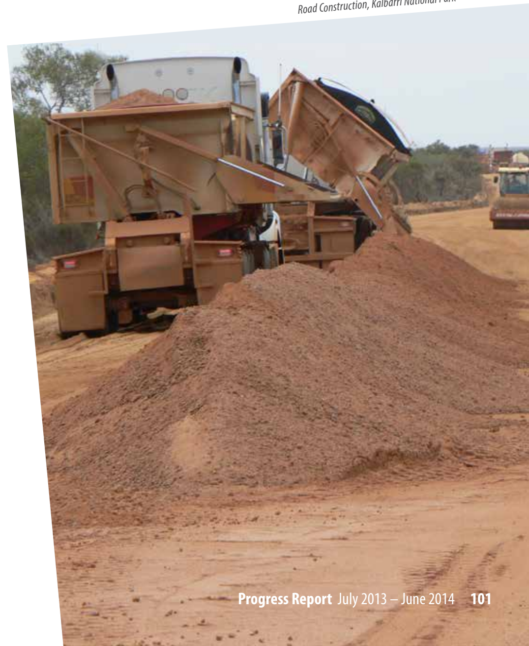
Road Construction, Kalbarri National Park
