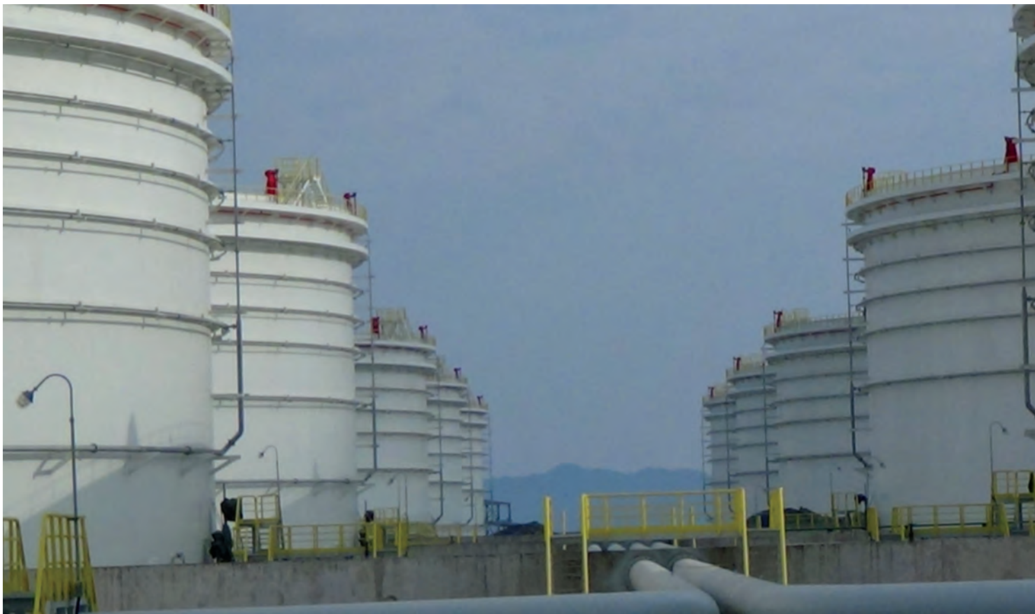
Tanks at the oil terminal in Kyauk Phyu Photo AOW
